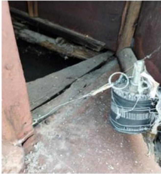
Figure 4: Grenade Installed in Door Entryway in Lachin District 40
